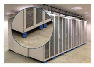
Patented Solution designed for Data Center protection against external vibrations:
